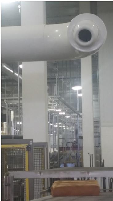
air movement helps employees feel more comfortable and by providing a cooling effect on the skin. Typically, designing to change the air from the floor to ten feet above the floor, six to ten times an hour in the summer, and four to six times an hour in the winter, is adequate. For workers who stay in a warm area constantly, such as slicing and packaging, spot cooling is a good way to provide economical comfort.
