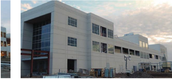
Use of architectural panels with the long dimension horizontal allowed for panelization consistent with the overall aesthetic, and allowed for pleasing joint and reveal locations without increasing material cost. Photo: The Austin Company/Northrop Grumman
