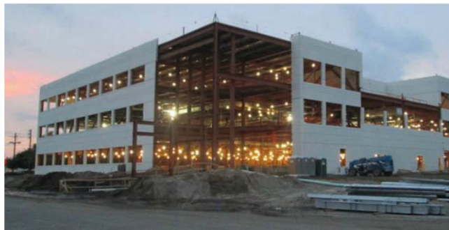
A structural steel framing grid was employed with an exterior cladding system comprising approximately 400 precast concrete panels. Photo: The Austin Company/Northrop Grumman
